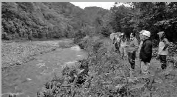
▶ 千走川左岸の決壊箇所を調査
